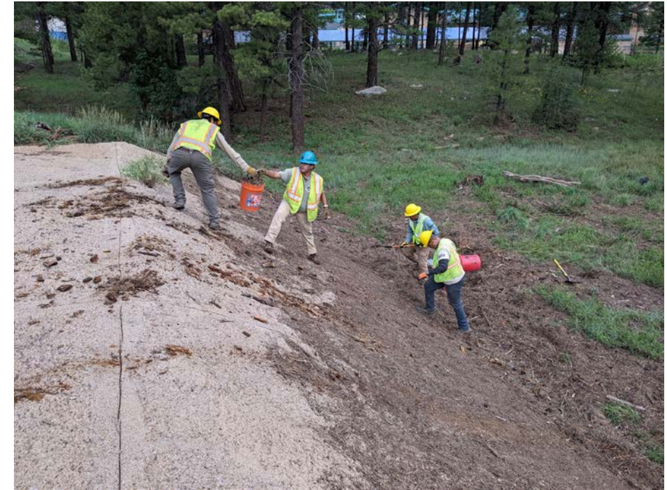
Ancestral Land crew cleaning detention basin near DeMiguel Elementary School
